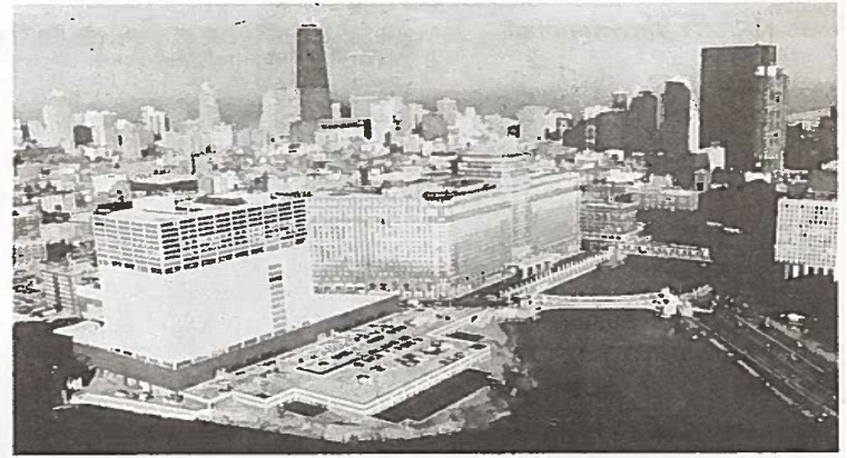
On the left, the Apparel Center which houses the 140,000 square foot ExpoCenter/Chicago, fashion show rooms and the Holiday Inn-Mart Plaza. To the right is the Merchandise Mart, the country's first wholesale furniture and fashion center. The Mart has 7½ miles of corridors on 97 acres of floor space (which would cover the entire Loop, if spread out) and occupies a square block at Wells and Kinzie Streets. Both buildings stand on Wolf Point, where the Chicago River branches to the North and South, and together they form a profitable wholesale marketplace for clothing, home and contract furnishings, and accessories.
