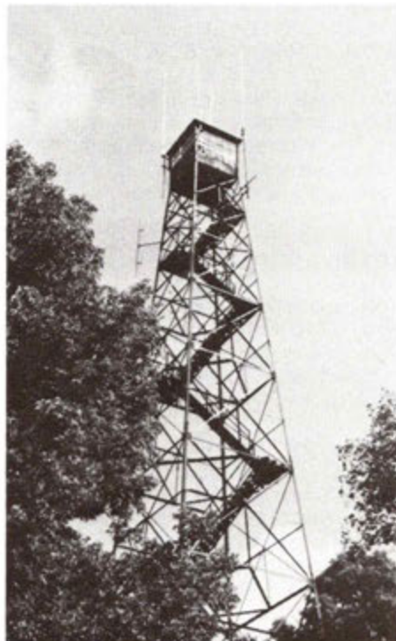
Array of CB, GMRS and Amateur antennas on the Holsclaw Hill fire tower.
