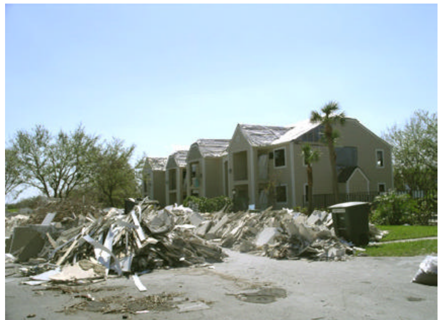
An apartment complex in Vero Beach after Hurricane Jeanne passed through. (Photo: Linda Konrad)
