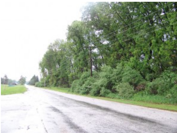
Storm damage by Oregon-Davis Schools
