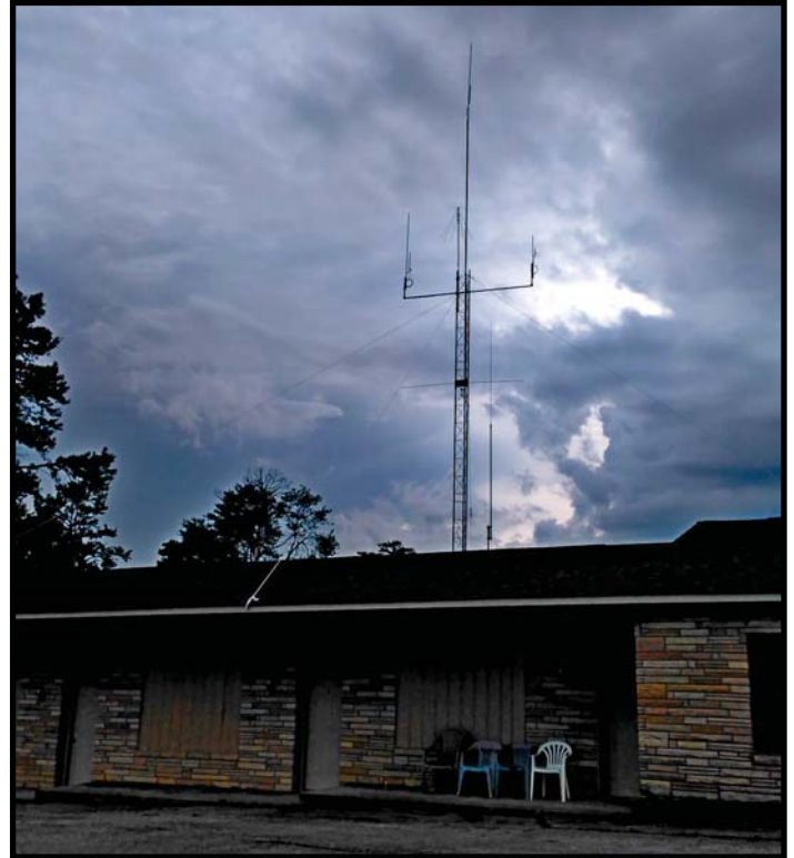
Antenna structure at the Starr Mountain REACT Headquarters/Mini-EOC
