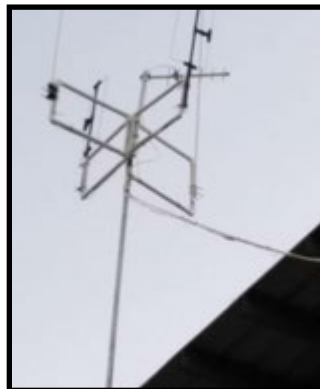
New antenna installation
